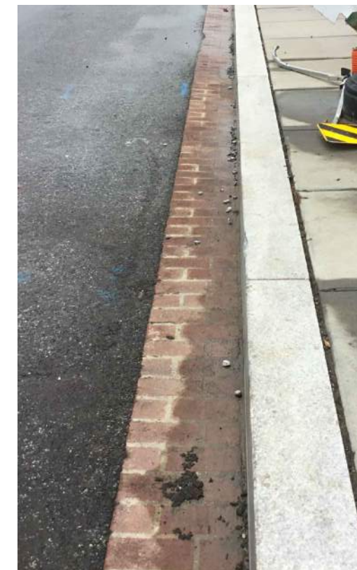
STONE CURB W/ BRICK GUTTER
